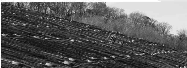
Temporary Rain Shed Cover
