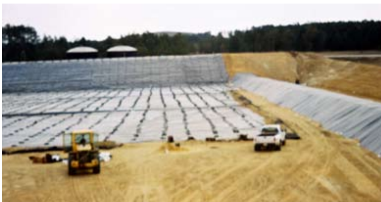
Interim Landfill Cover
